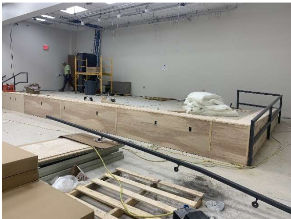
Miscellaneous Carpentry – Auditorium Stage
