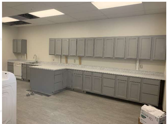
Homemaking Classroom - Casework Installation
