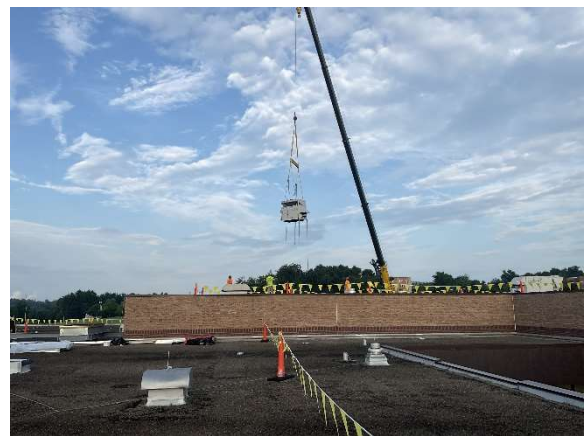
RTU Crane Lift - Roof
