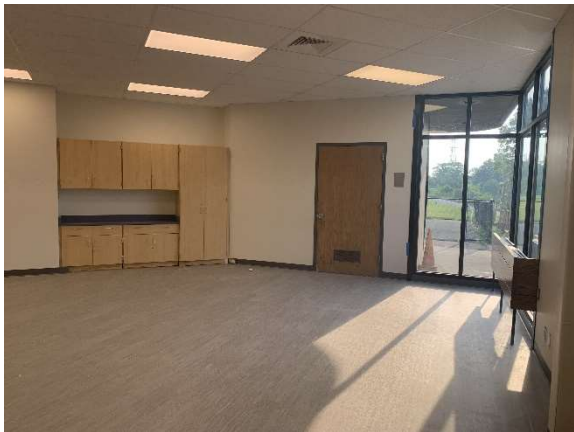
New Classroom Casework
