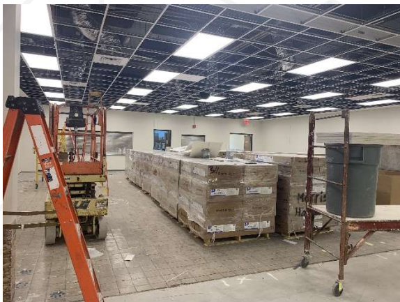
Ceiling Grid - Cafeteria
