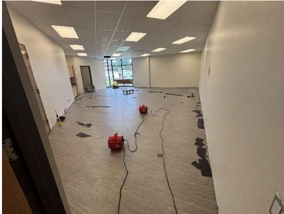
Flooring Installation – 20 Pod Classroom
