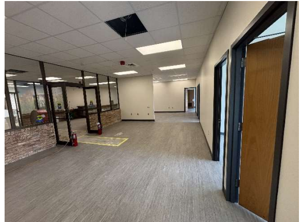
Flooring Installation – Admin Offices
