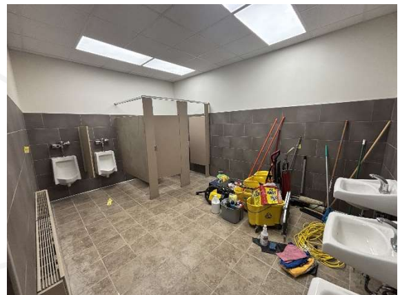
Partition & Fixture Reinstallation – Restrooms
