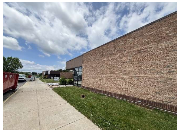
Brick Cleaning & Sealing – Exterior
