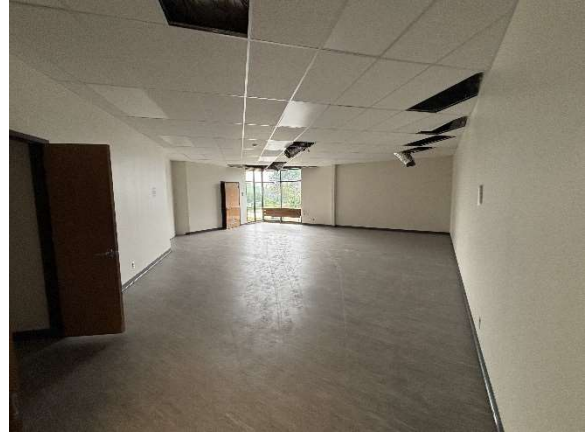
Ceiling Tile Installation – 80 Pod Classroom
