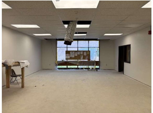
Ceiling Tile Installation – Library
