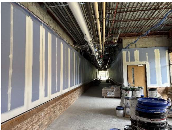
Taping & Finishing – 40 pod to 20 pod Corridor
