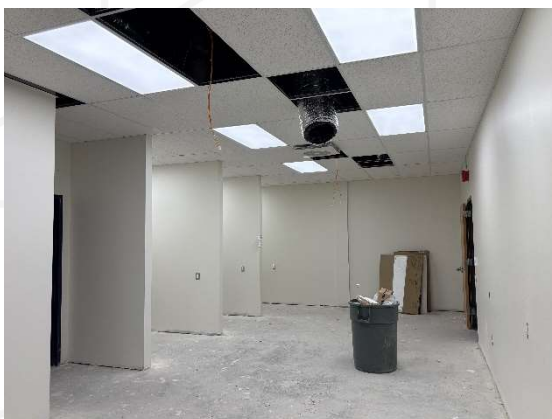
Ceiling Tile Installation – Nurses Office
