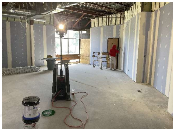
Taping & Finishing – 20 pod classroom
