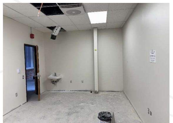
Ceiling Tile Installation – Nurses Office
