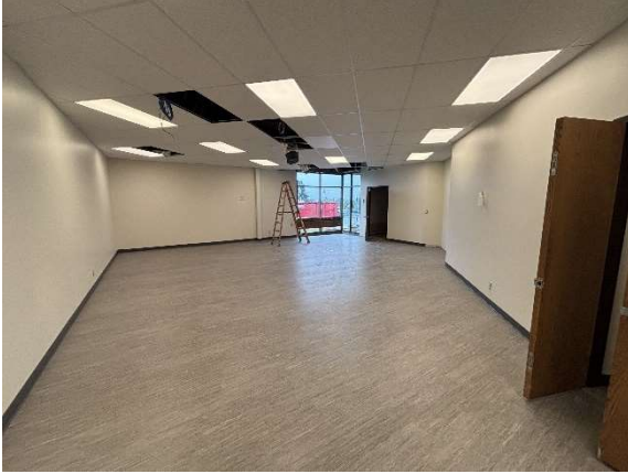
Ceiling Tile Installation – 80 Pod Classroom
