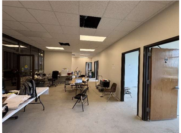
Ceiling Tile Installation - Admin
