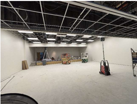
Painting & Ceiling Grid Installation – Auditorium
