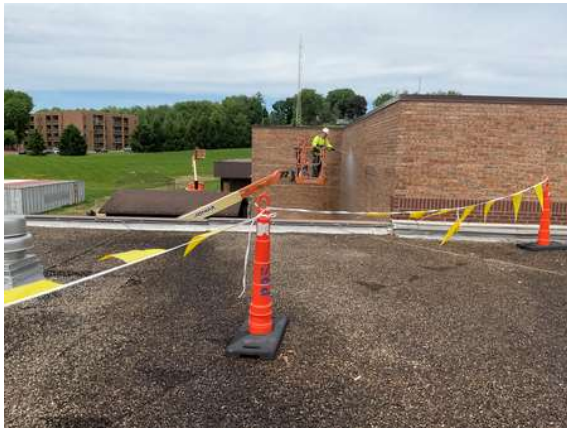
Brick Cleaning & Sealing
