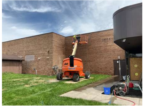
Brick Cleaning & Sealing
