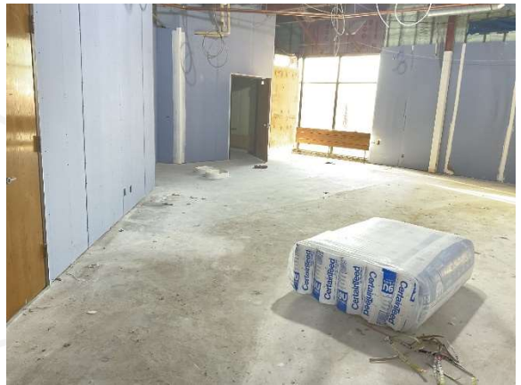
Drywall Installation – 40 Pod Classroom
