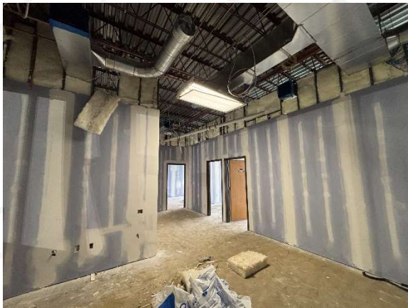
Taping & Finishing – Admin Office
