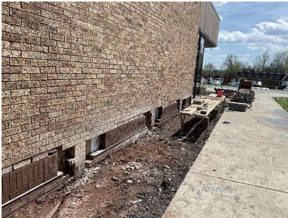
Brick Restoration – Main Entrance
