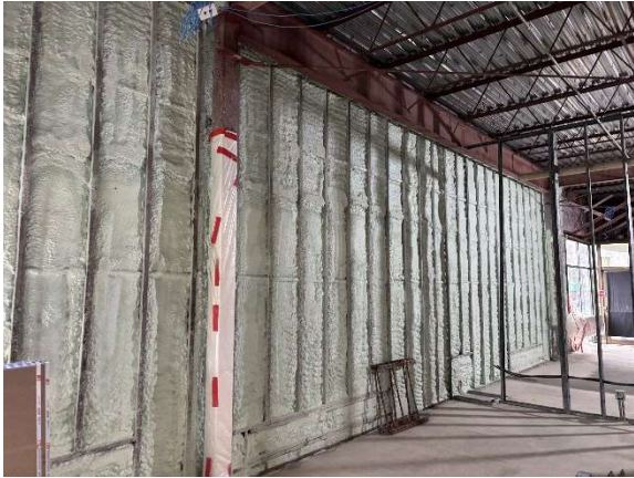
Spray Foam Insulation – 80 Pod Classroom
