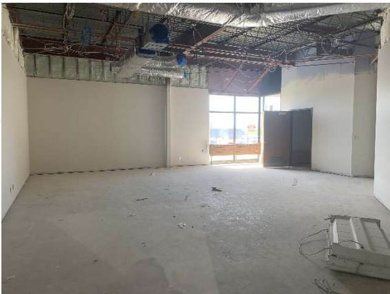
Painting & Ductwork – 80 Pod Classroom
