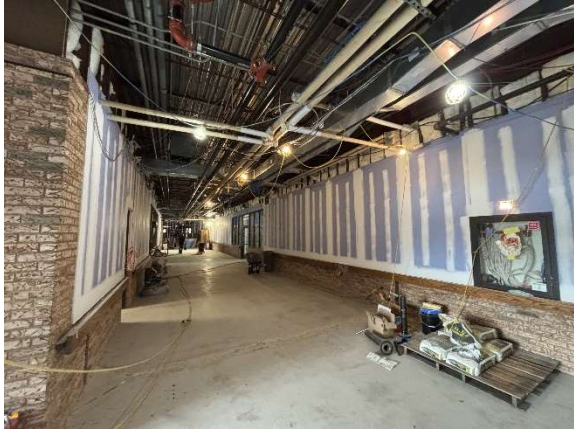
Taping & Finishing – Admin Corridor
