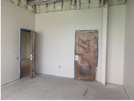
Painting – Admin Office
