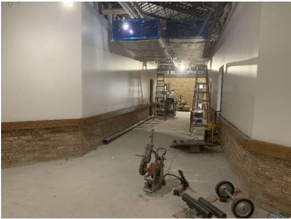
Painting – 80 Pod Corridor
