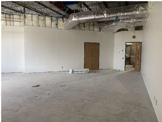
Painting & Ductwork – 80 Pod Classroom
