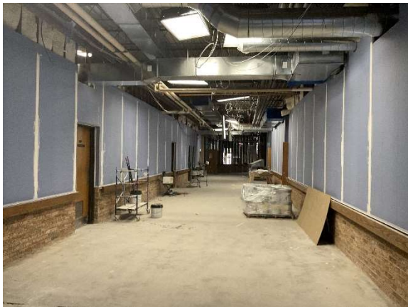
Drywall Installation – North Corridor
