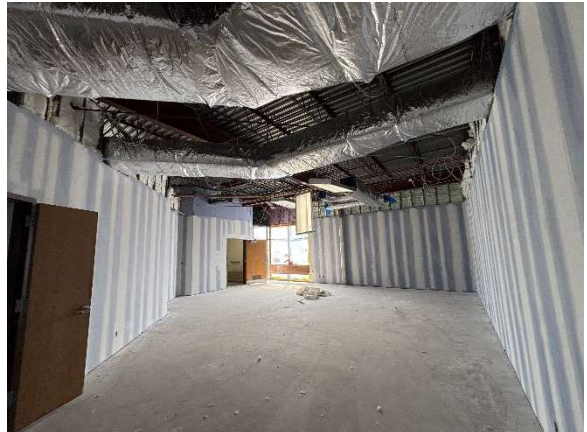
Drywall Taping & Finishing – 80 Pod Classroom
