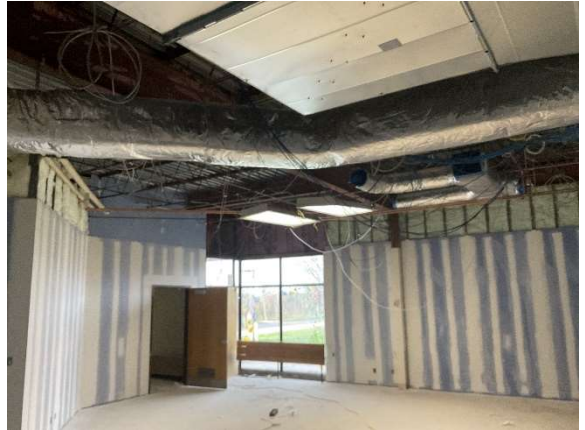
Taping & Finishing – 60 Pod Classroom
