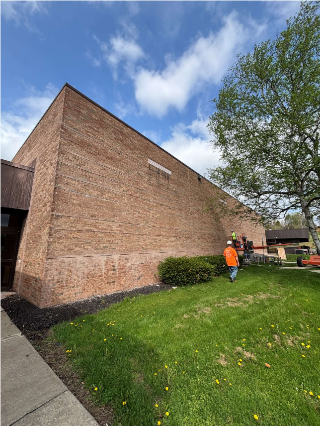
Masonry Restoration Progress
