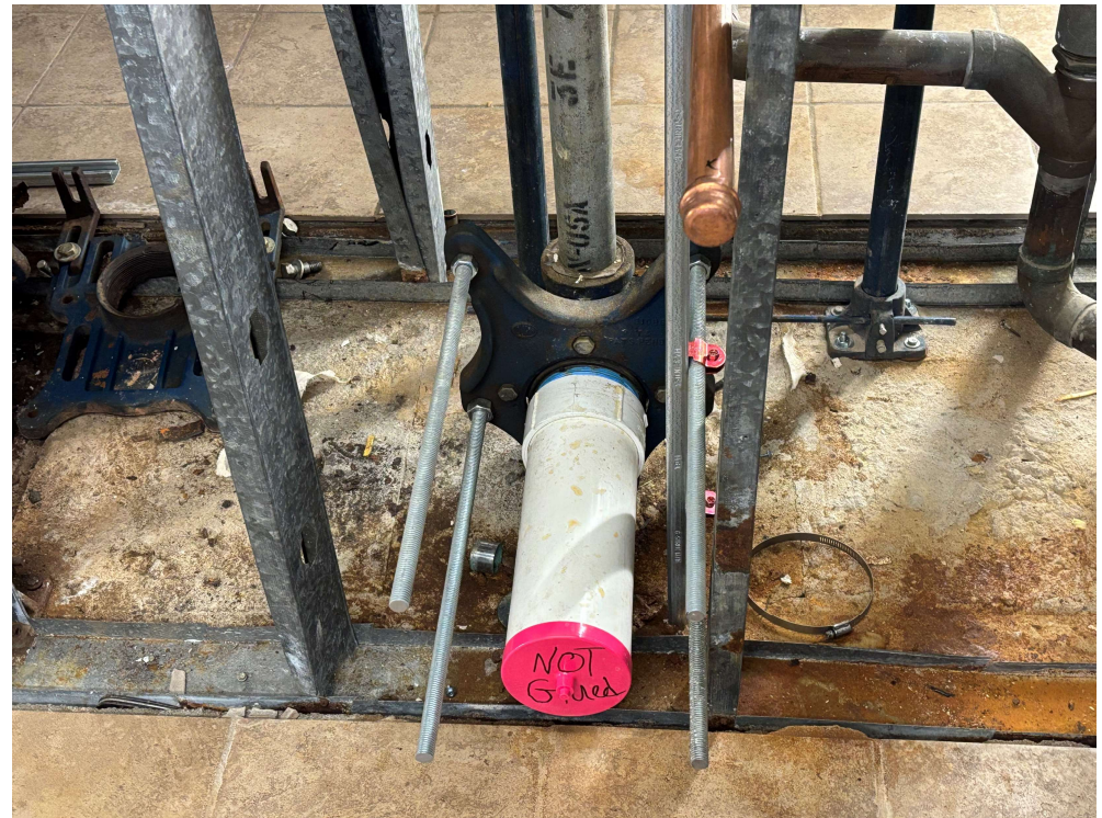
New Restroom Plumbing
