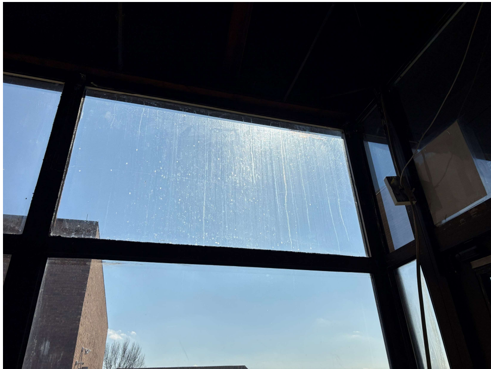
Existing Window Condition
