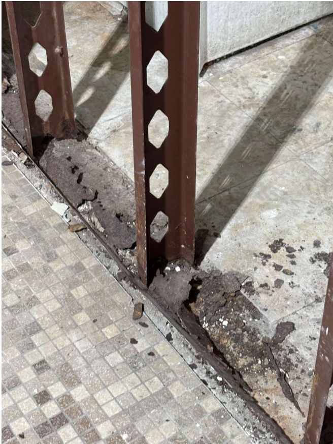
Existing Metal Framing Replacement
