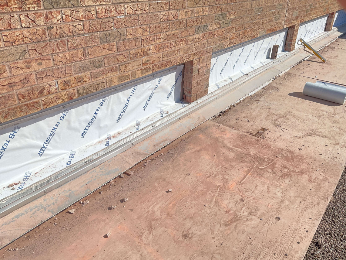
New Masonry Flashing
