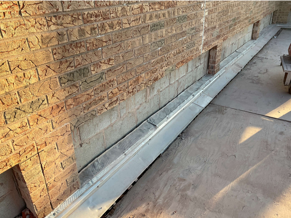
Existing Masonry Cavity
